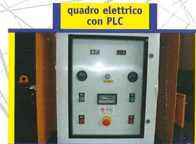
electric cabinet with PLC
